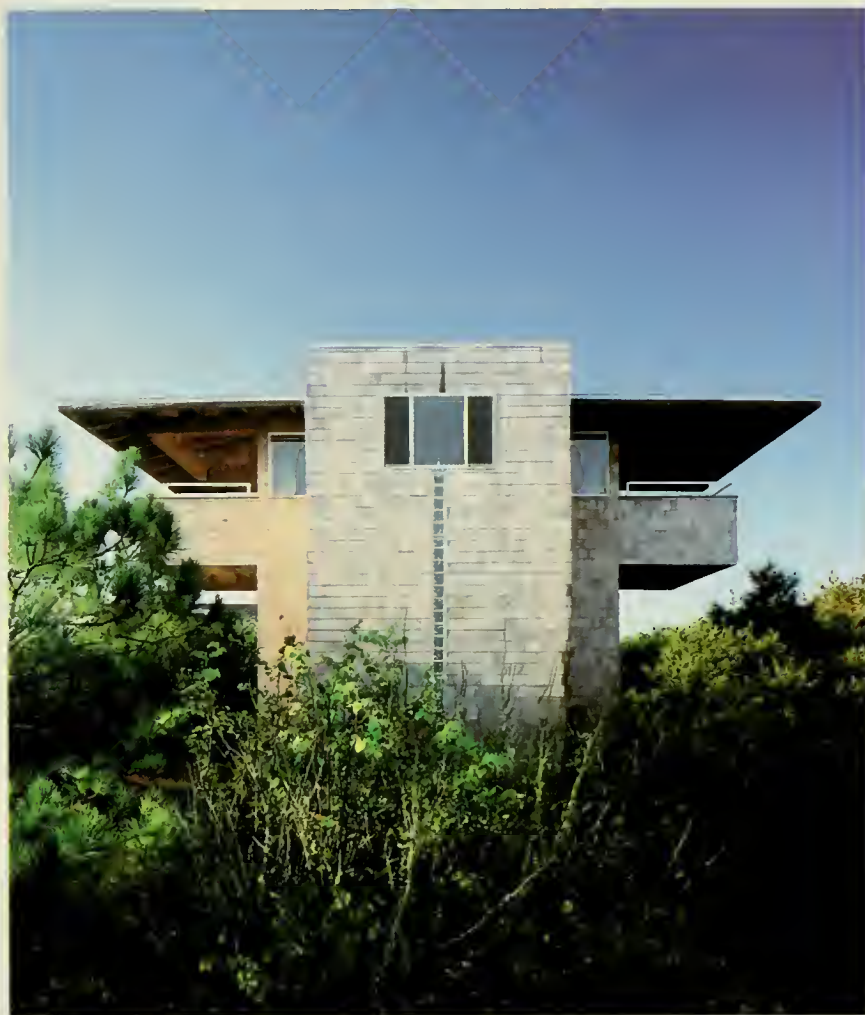
Drysdale Residence, Atlantic Beach
